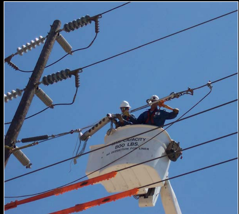
Installation in progress
