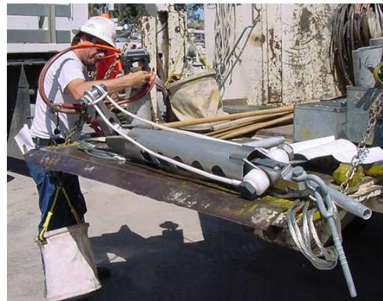
Figure 4: The SLiM device prepared for installation.
