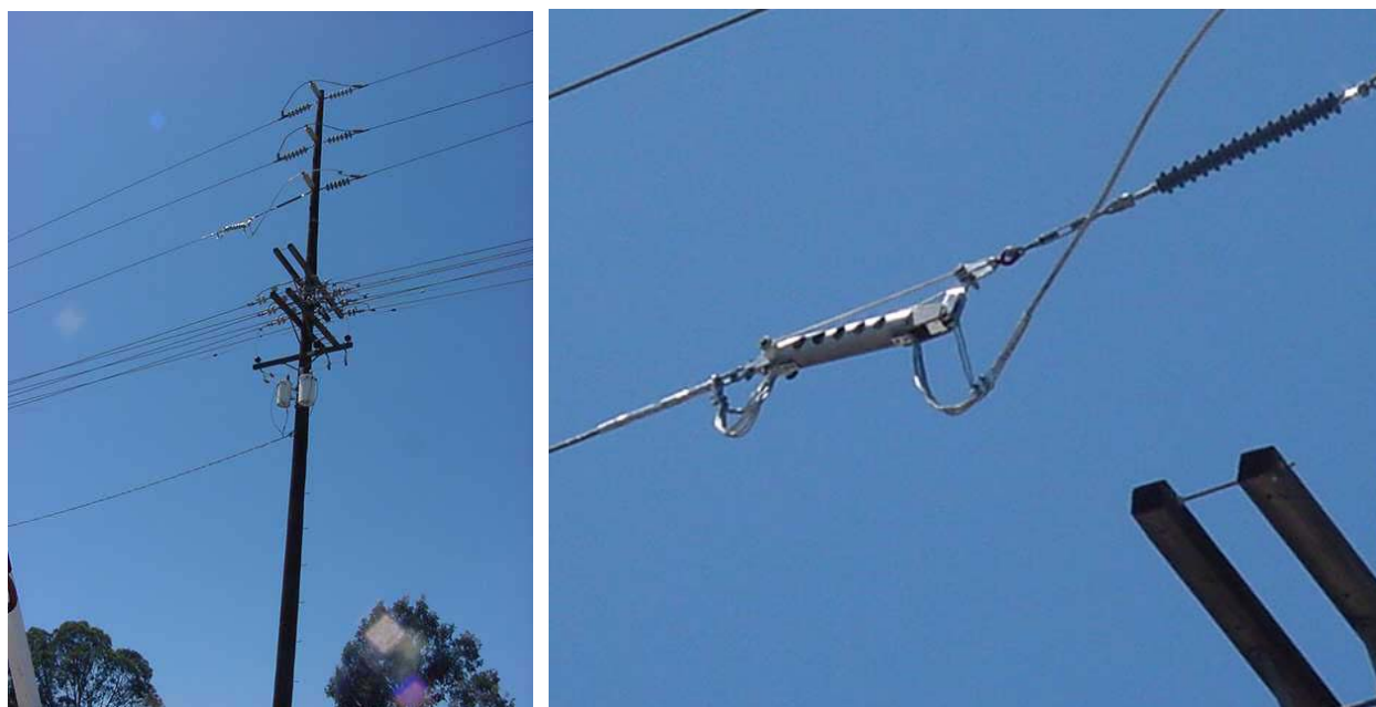
Figure 5: Completed installation of the SLiM device.
